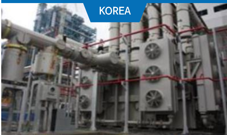
345KV 690MVA Dangjin Thermal Power plant
