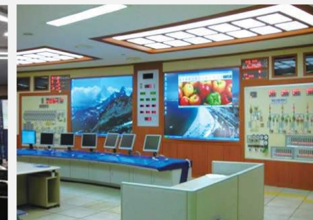
Ilsan Cogeneration 2 Power Plant S/T main control system ('13)
