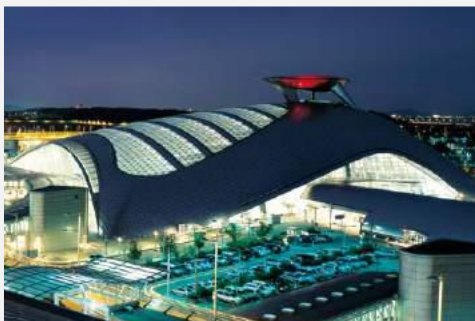
Incheon International Airport Terminal 2 Power Control System ('13 ~ '17)
