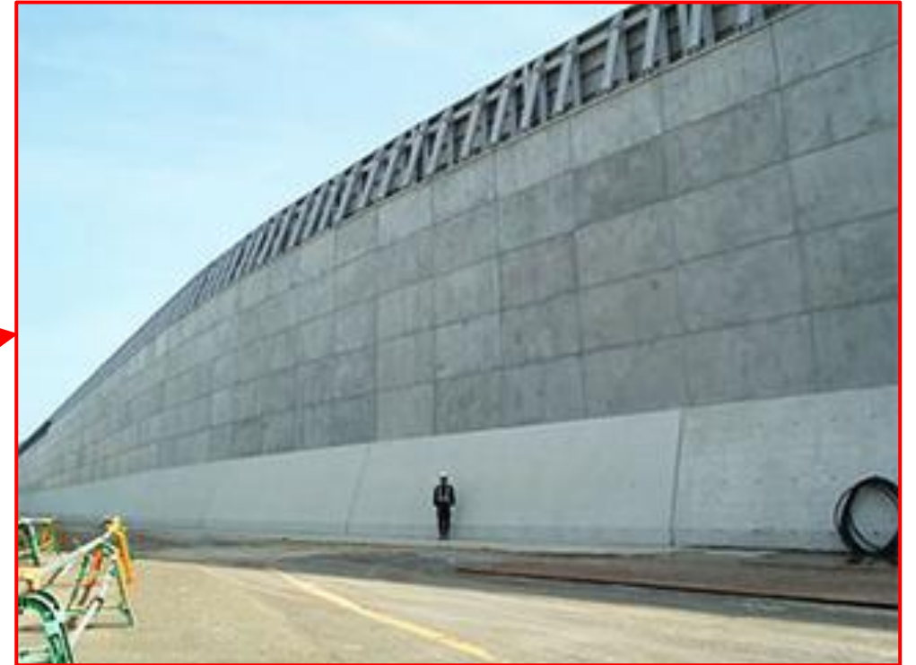
Tsunami Protection Wall (22m above sea level, 1.6km long) (16m above ground level)
