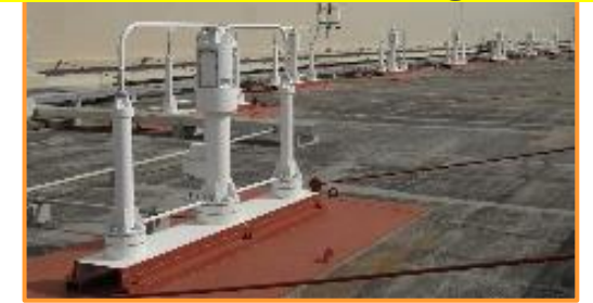
Oceanographic Radar measures sea surface current velocity
