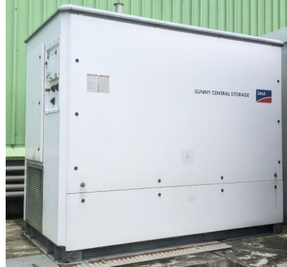
SMA PCS (grid following & forming)
