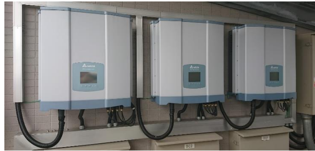
PV Inverter 1 PV Inverter 2 PV Inverter 3
