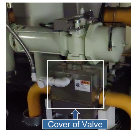
Fig.2 Valve Cover
