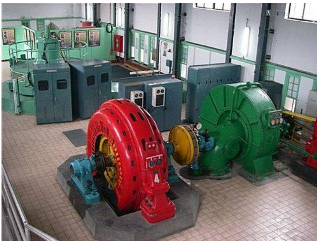
View of the Generators and water turbine
