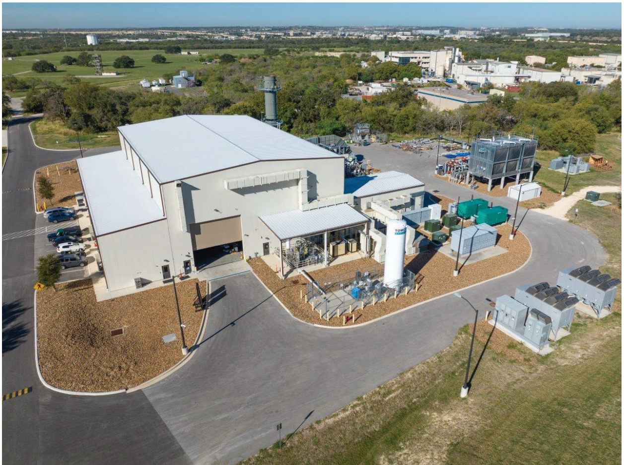
Aerial View of Supercritical Transformational Electric Power (STEP) 10 MWe Pilot Plant
