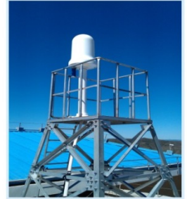
lightning Detecting Station
