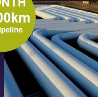
1.4m dia pipe @100bar
