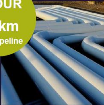
1.4m dia pipe @100bar
