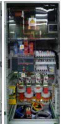
Battery power Incoming panel
