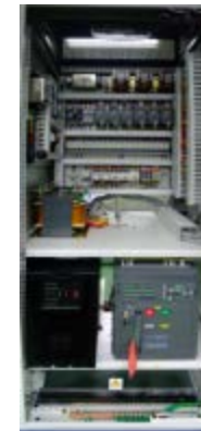
Main control panel
