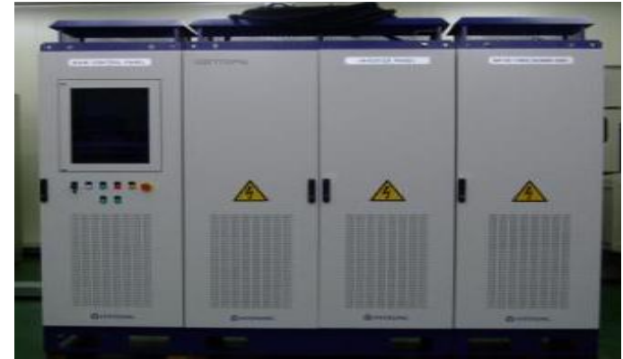
1MW ES-PCS Panel
