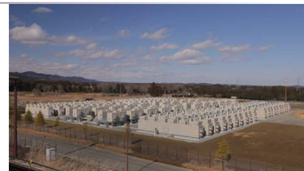
40MWh Li-ion Storage System (Tohoku Electric Company)
