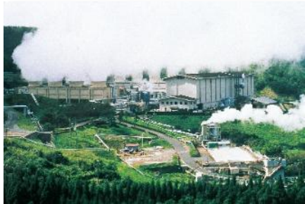
Geothermal Power Plants
