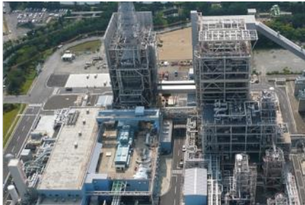
Integrated Coal Gasification Combined Cycle (IGCC) Power Plants
