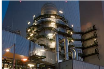
Environmental Plants SCR (DeNO x ) Systems / Flue Gas desulfurization
