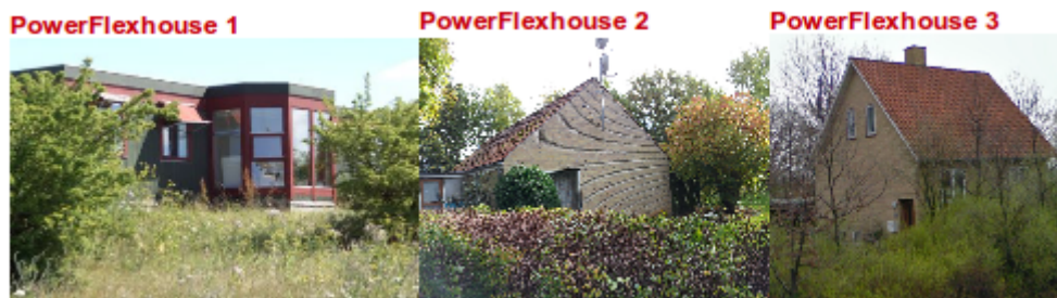
Figure 1: Three PowerFlexHouses in SYSLAB
