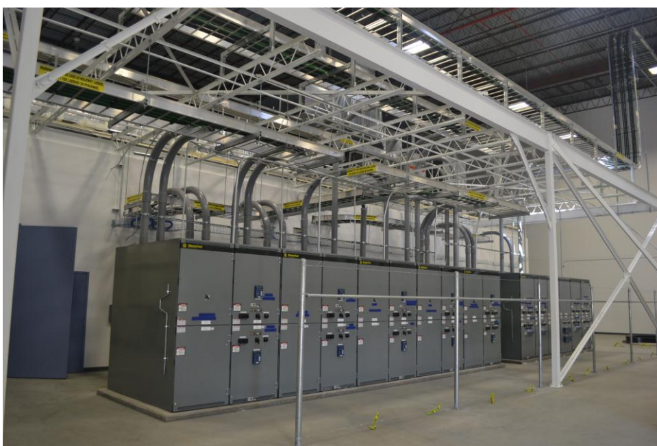
EGRID 5 kV and 25 kV Switchgear and indoor testing space
