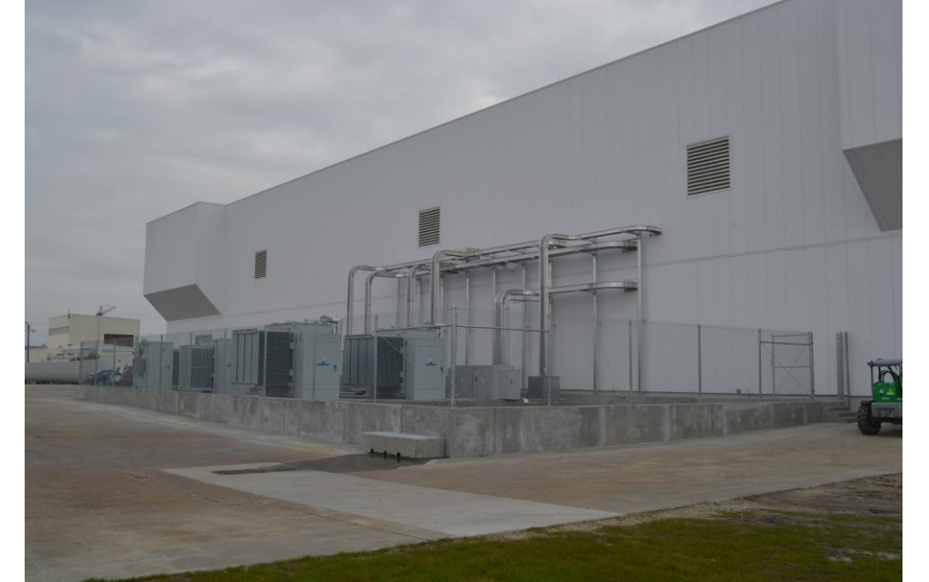
Outdoor Transformer Yard and Reinforced Concrete Testing Area
