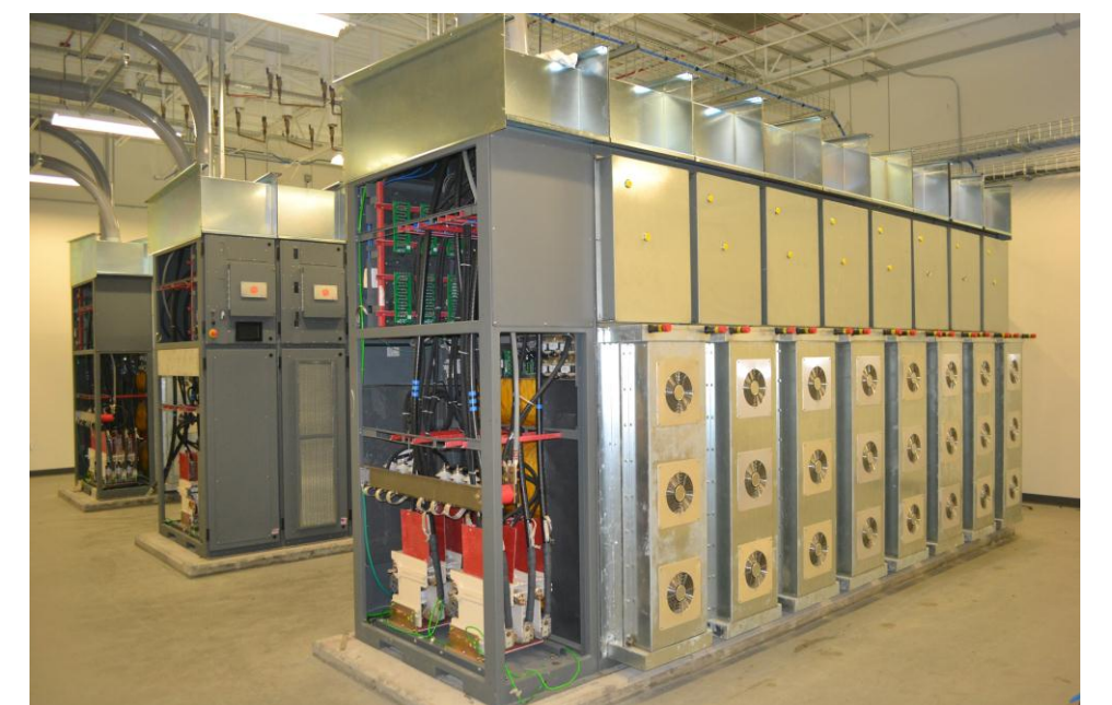
Power Amplifier Room with 4 separate amplifier cabinets
