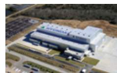
HYUNDAI POWER TRANSFORMERS USA
